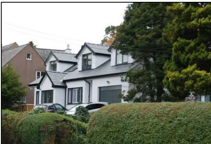
Dormers out of scale to local context
