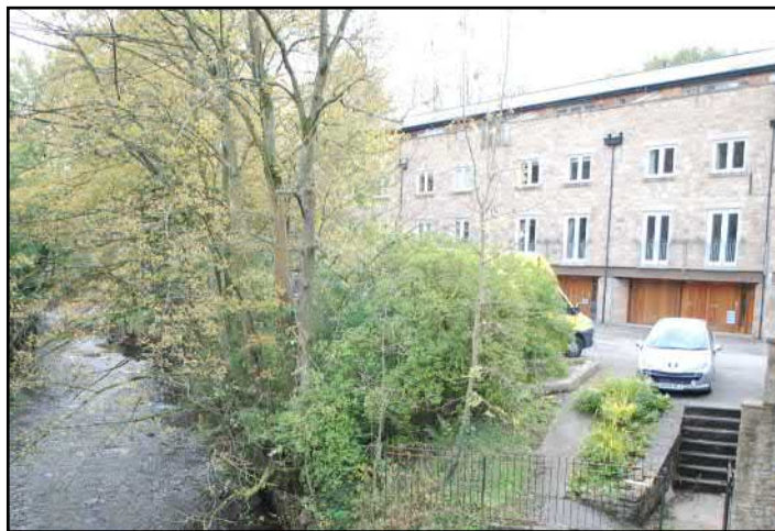
Good example of adopting more resilient ground floor uses (parking)
