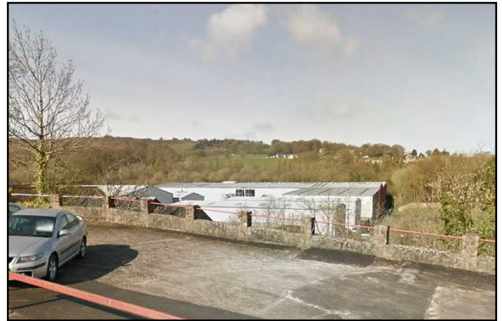
Example of poorly screened large scale development, seen from Buxton Road
