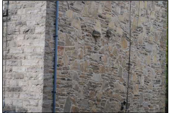
Example of different uses of gritstone. Simple downpipes
