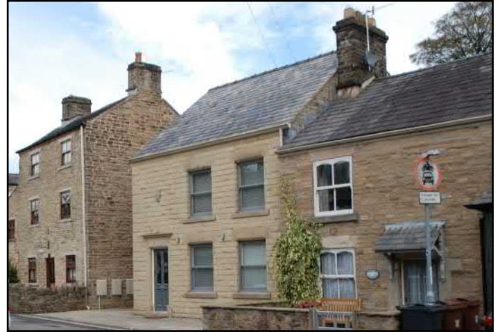
Sympathetic solid and void ratio, glazing details, door fittings and colour tones. Closely matched stone colour
