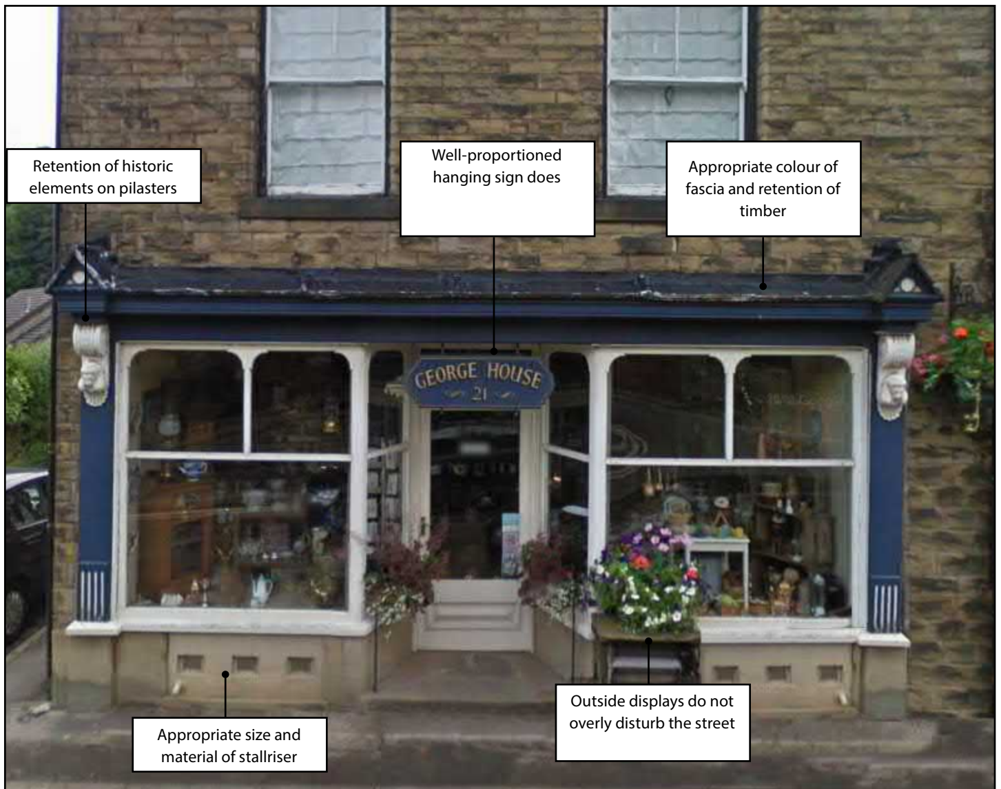
Figure 34: A good example of a traditional shop-frontage
