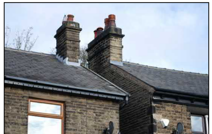
Chimneys are common
