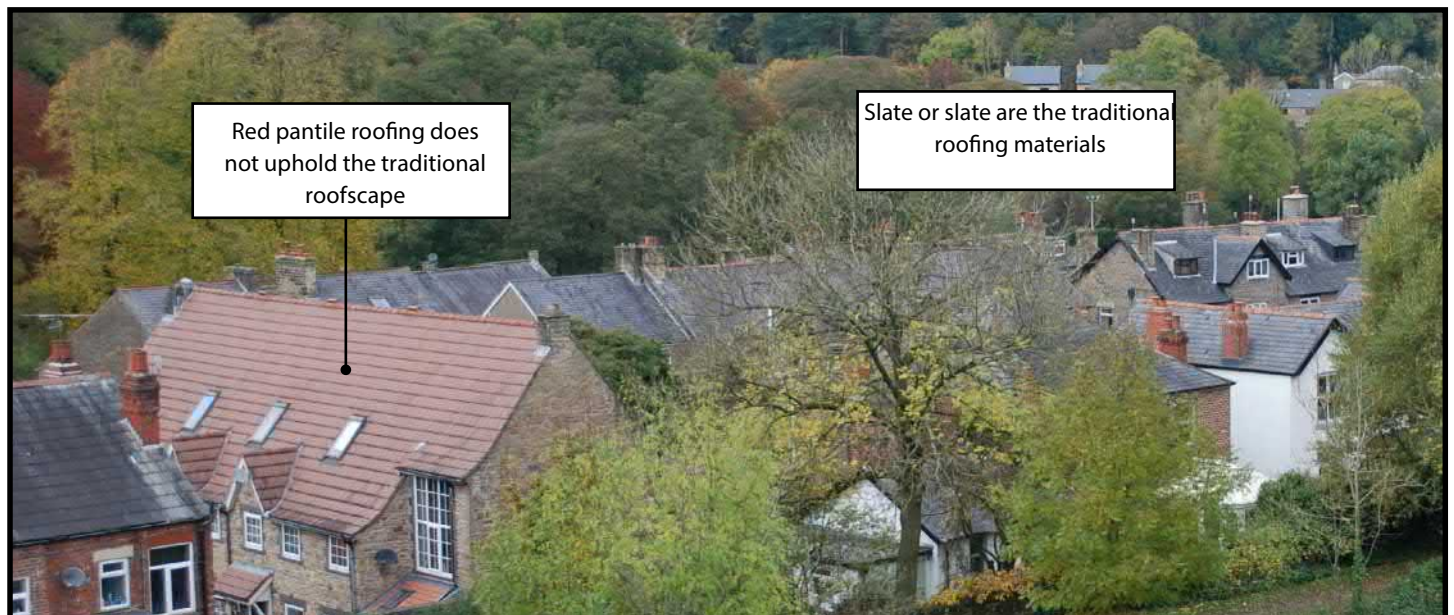
Figure 38: Code BM3 Roofing
